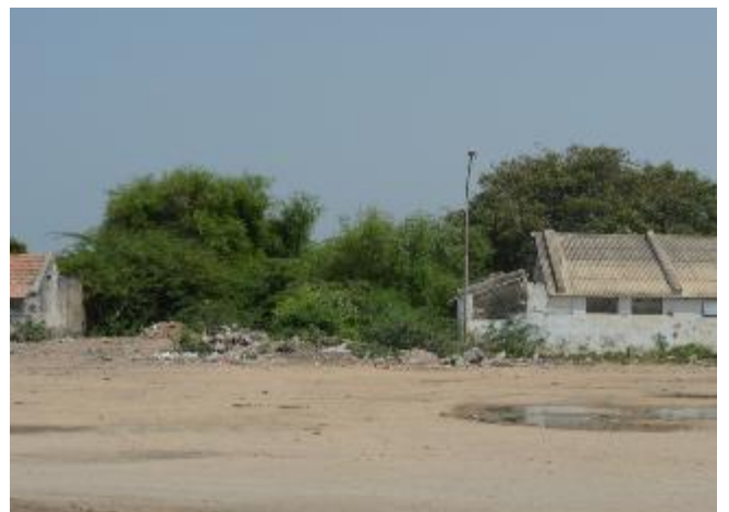
Concrete pile and dense vegetation between houses (Cl. C)
