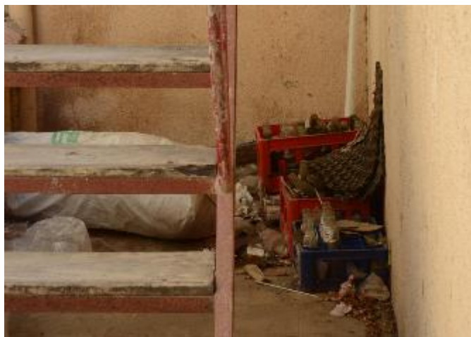
Pile of occasionally used items (Cl. D)
