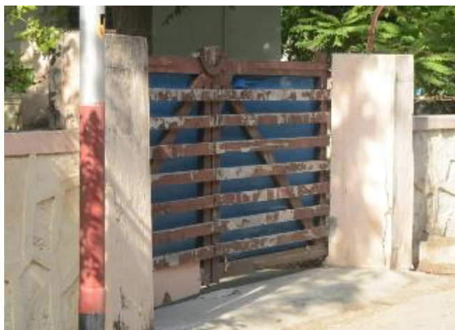
Main gate having space on lower side (Cl. D)
