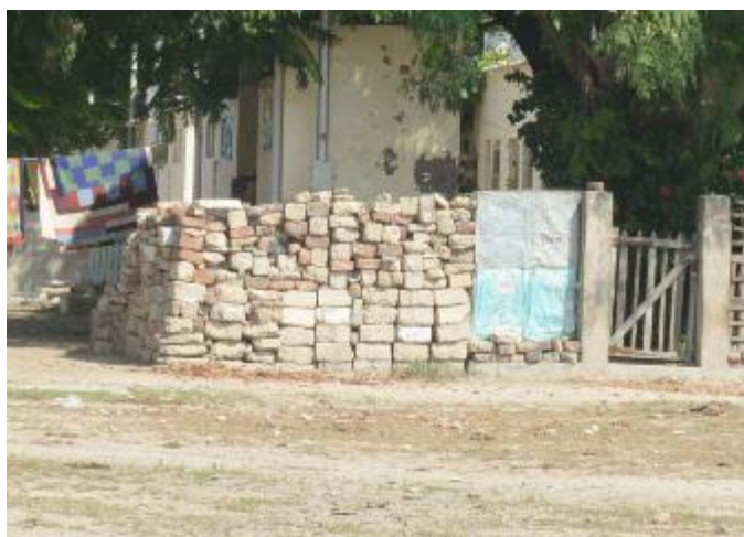
Non-plastered thick wall of rocks (Cl. D)
