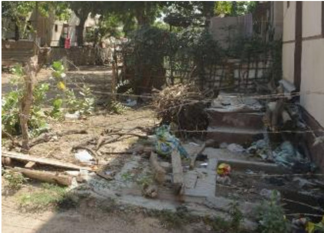
Poorly piled firewood and junk (Cl. C)
