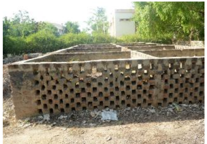
Constructions having pores and gaps (Cl. A)
