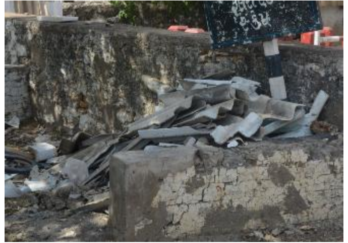
Poorly arranged pile of sheets (Cl. A)
