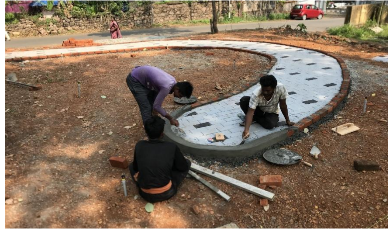
Figure 17. Walkway were build using interlock blocks
