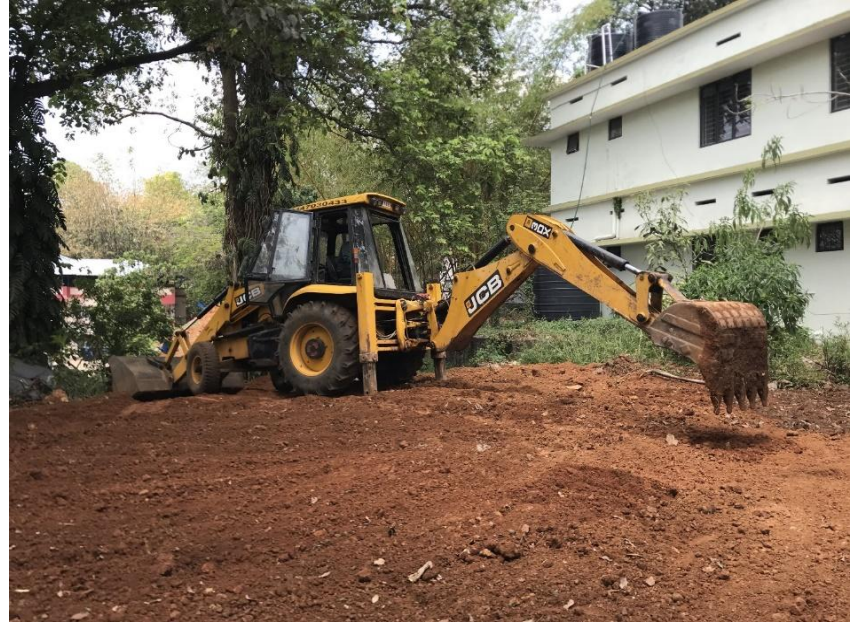
Figure 7. Site leveling using machineries
